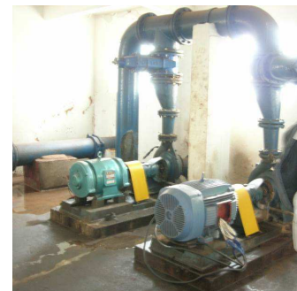
Unidades de recalque: 1x75CV + 2 x 50 CV (planilha ref. 1), ou 1 x 70CV + 1 x 50CV + 1 x 40CV (planilha ref. 2)
